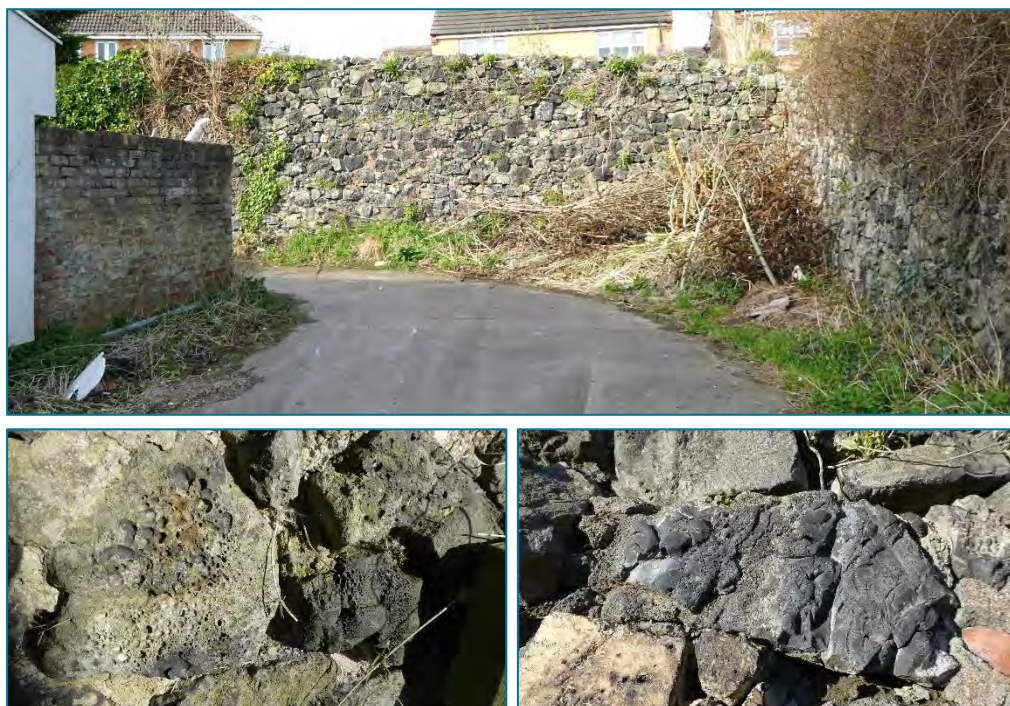
Top: Remains of southern boundary wall of the [Q] Middleton Iron Works, bordering the back lane to Killinghall Row, Yarm Road, the first houses to be built for the increasing workforce. It is mainly constructed from slag with a few red brick pinnings in between. Smelting is the process of applying heat and a chemical reducing agent to an ore to extract a desired base metal product. As most ores are impure, it was necessary to use limestone, which was brought in from Weardale, to remove the accompanying rock gangue as slag 101 . This wall is now the only survivor of the iron works site (Photo © Gaby Rose, March 2024). Bottom: Details of slag pieces. (Photos © Gaby Rose, February 2025)
