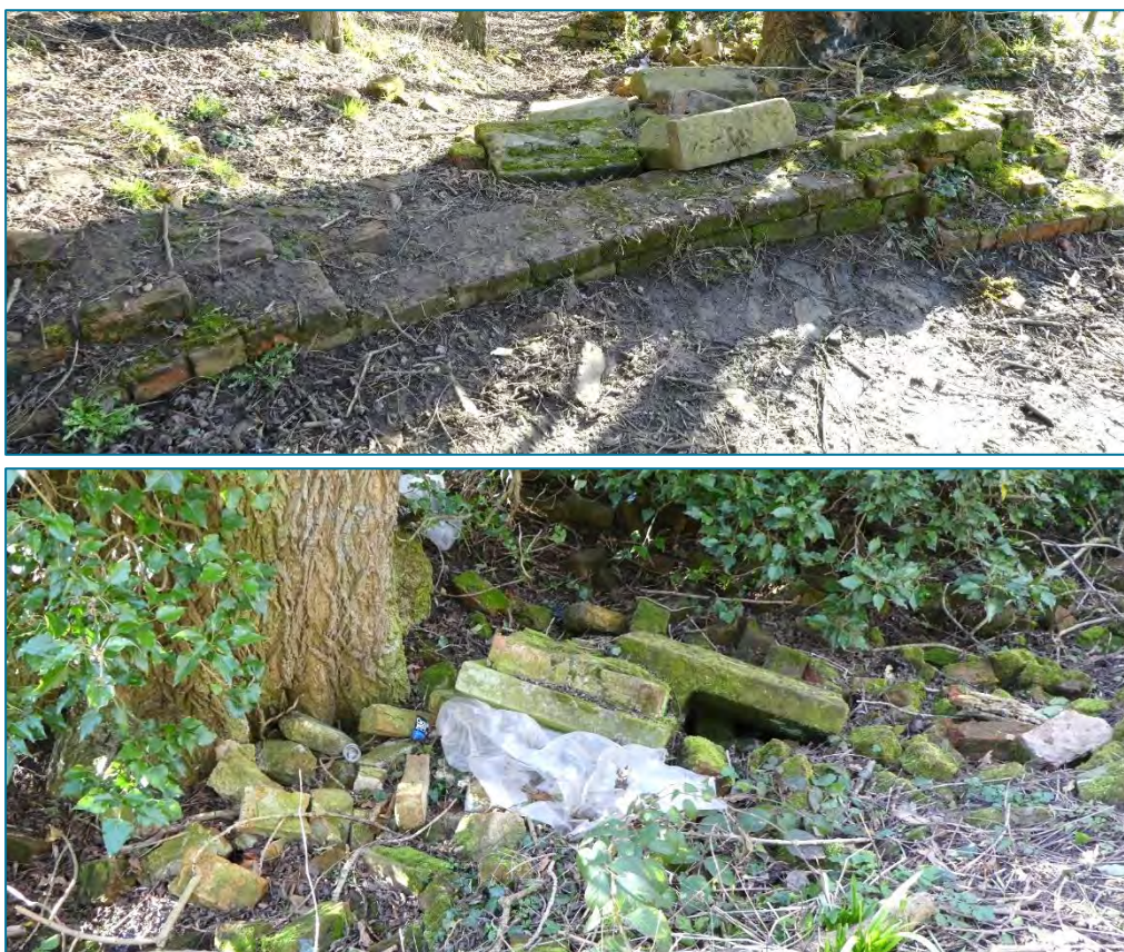
Top: End section and terminal pier (right) of former reservoir embankment walling that has been destroyed by vandals. Bottom: Discarded rubbish, bricks and stone cappings opposite the dismantled walling. (Photos © Gaby Rose, February 2025)
